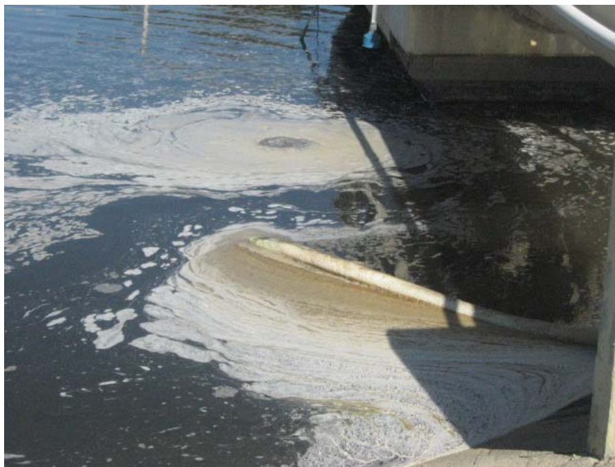
Photo 5: Brown scum on surface of effluent pump station wet well holding pond.
