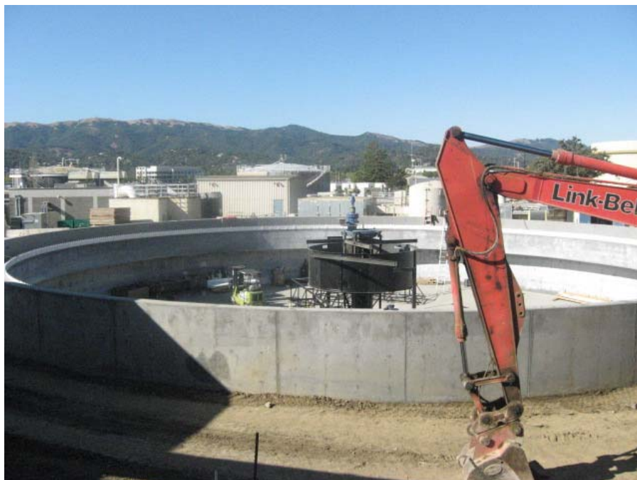
Photo 2: Primary clarifier under construction (looking westerly).
